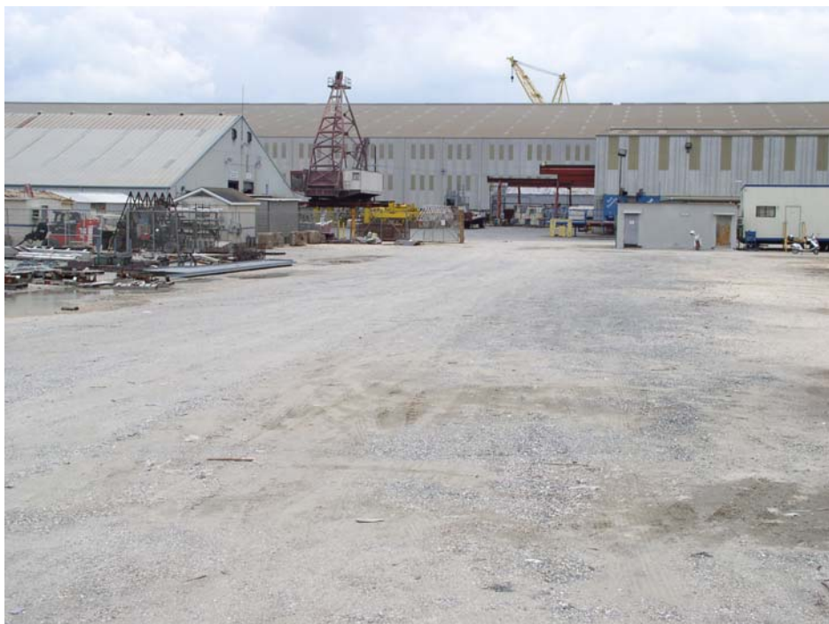
Receiving Area After
