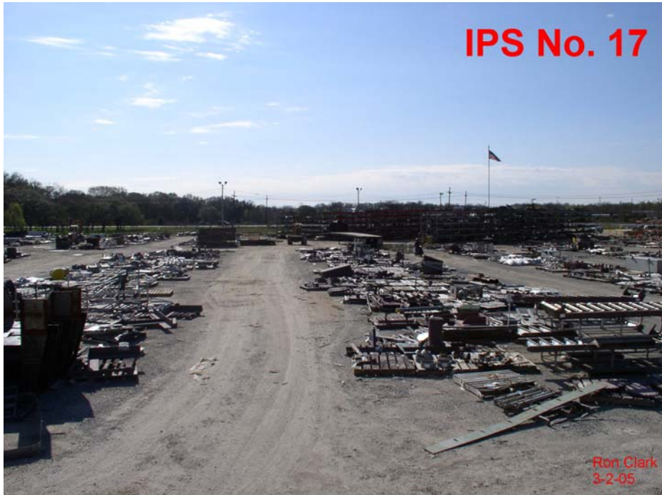
Storage Area Before
