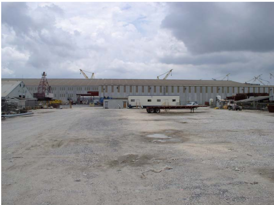
Lay Down Area After
