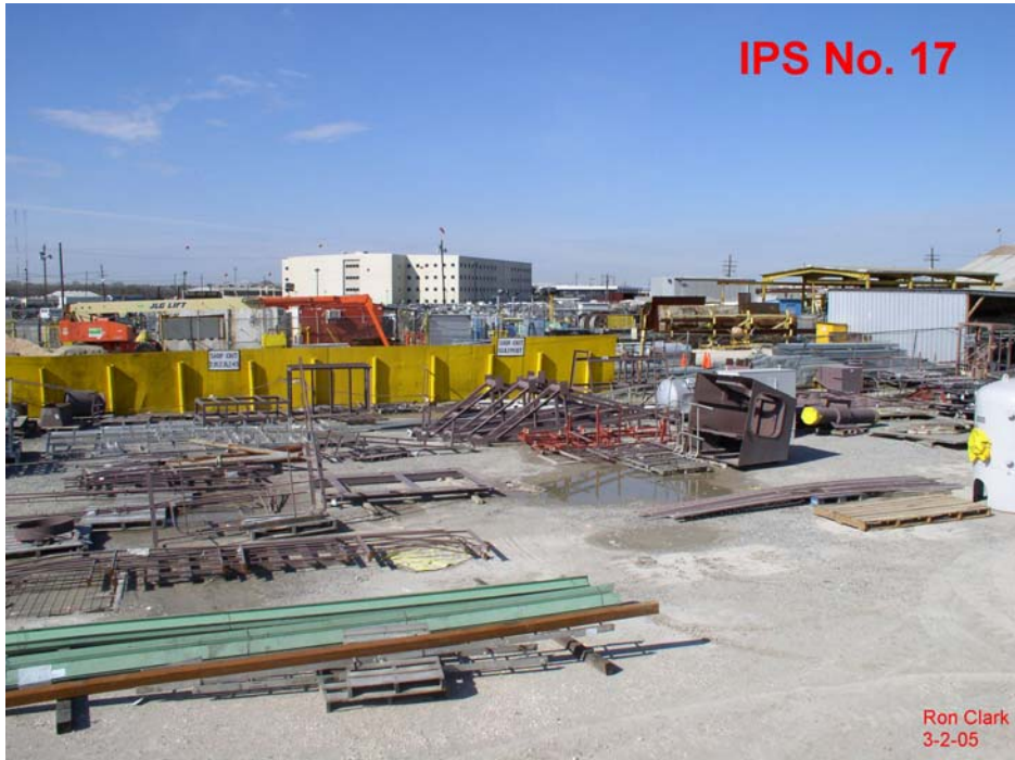
Lay Down Area Before
