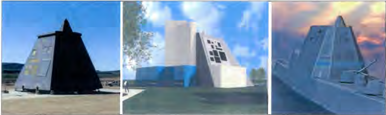
Figure 2 – DDG 1000 Composite Structures: the Integrated Deckhouse Test Article (IDHTA), Wallops Island Surface Combat Systems Center Test Facility, and the DDG 1000 composite deckhouse and hangar
