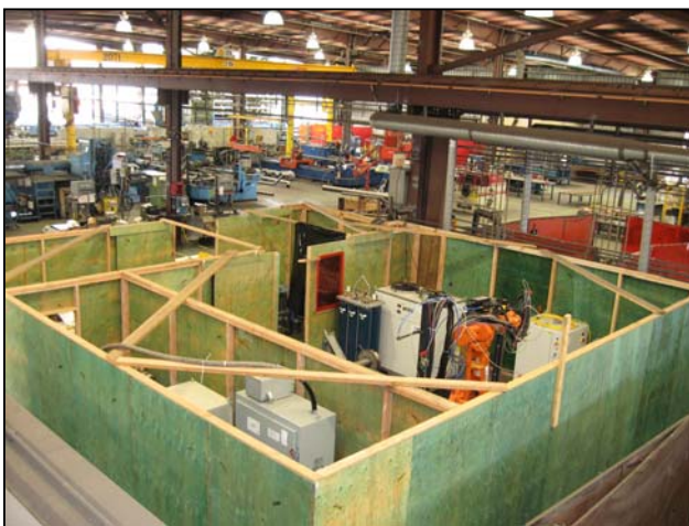
Figure 18. Aerial view of the hybrid pipe welding station and the safety enclosure installed in the GD NASSCO pipe shop.
