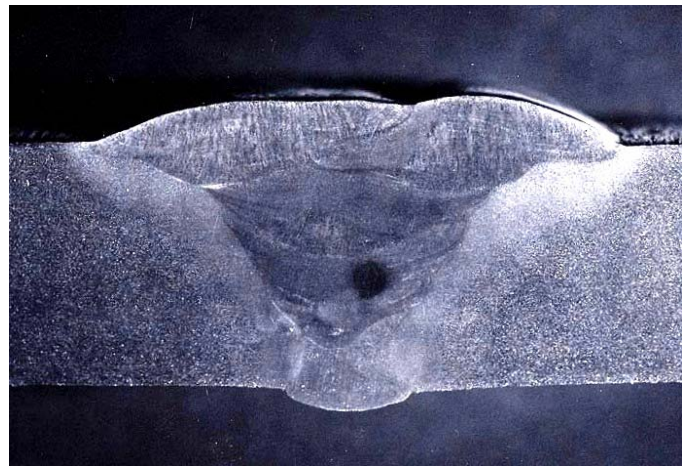
Figure 9. Cross section of conventional multipass pipe weld with 12.7 mm (0.5 in) thickness (courtesy GD NASSCO).
