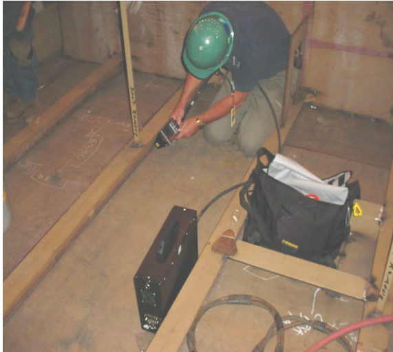
Figure 10 Unit in use
