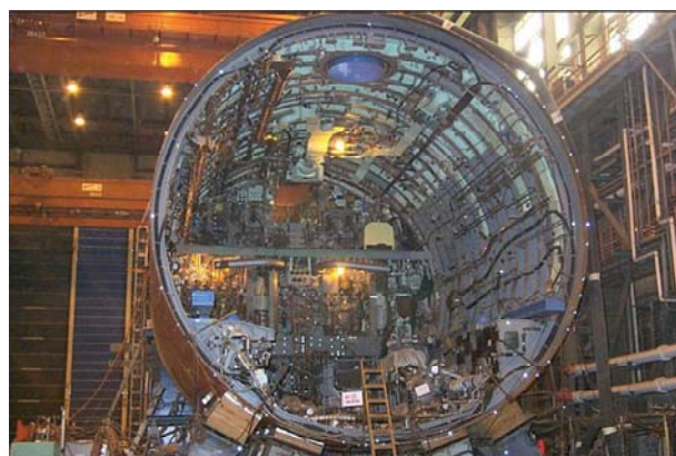
VCS cylinder outfitting during construction at Electric Boat.
