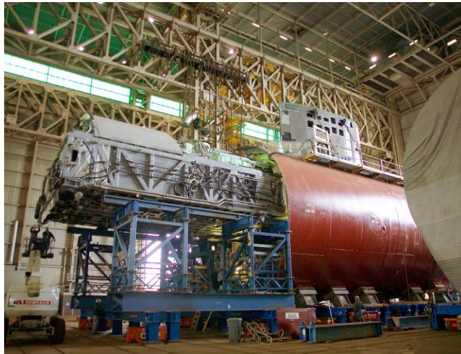
VCS Cylinder Outfitting During Construction at Electric Boat
