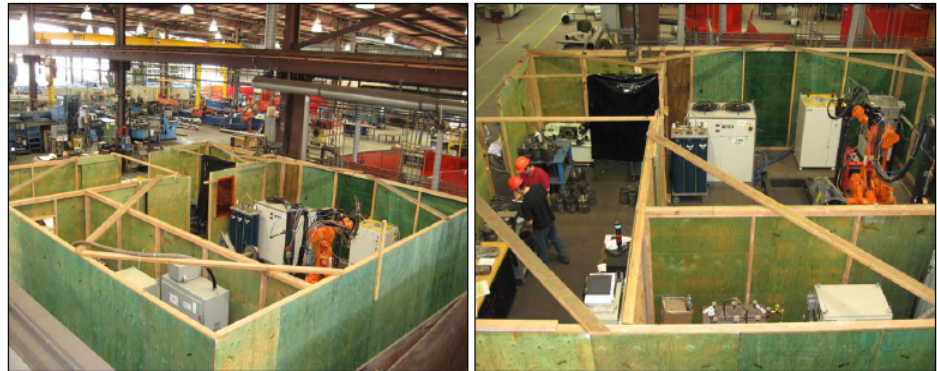
Aerial Views of the System Installed in GD NASSCO Pipe Shop.
